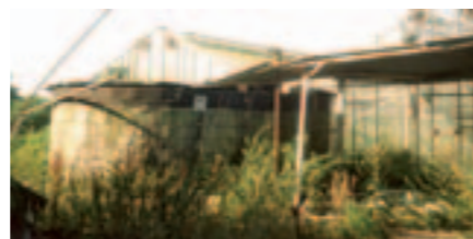
TOP: THE BOILER HOUSE BELOW: THE 6,000 GALLON WATER TANK
